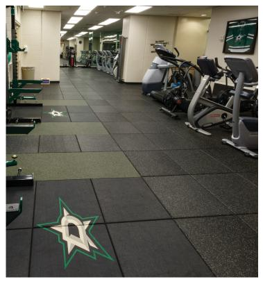
the shock of heavy impacts, protecting both athletes and the subfloor from potential damage. The modular design of the tiles allows for easy installation, repair, and replacement. Moreover, the slip-resistant surface ensures professional athlete safety during intense workouts. By creating a training environment that prioritizes safety, functionality, and performance, the Dallas Stars demonstrate their dedication to providing their athletes with the resources necessary to excel in their sport.
